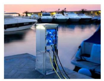
Figure 1. Marine-style pedestal with socket outlets
